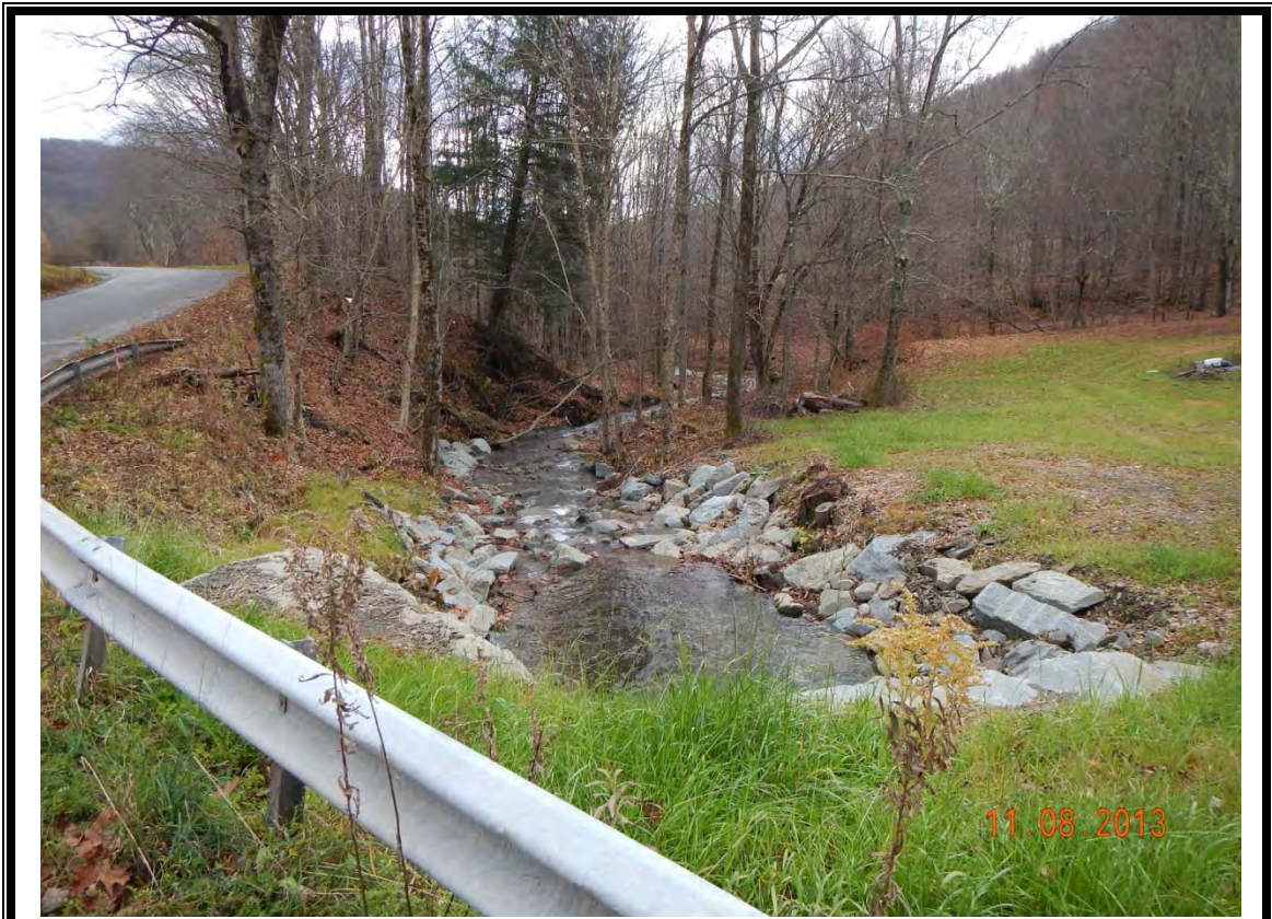
Photo 5: Looking downstream from Baxter Brook Road at plunge pool and step pools.
