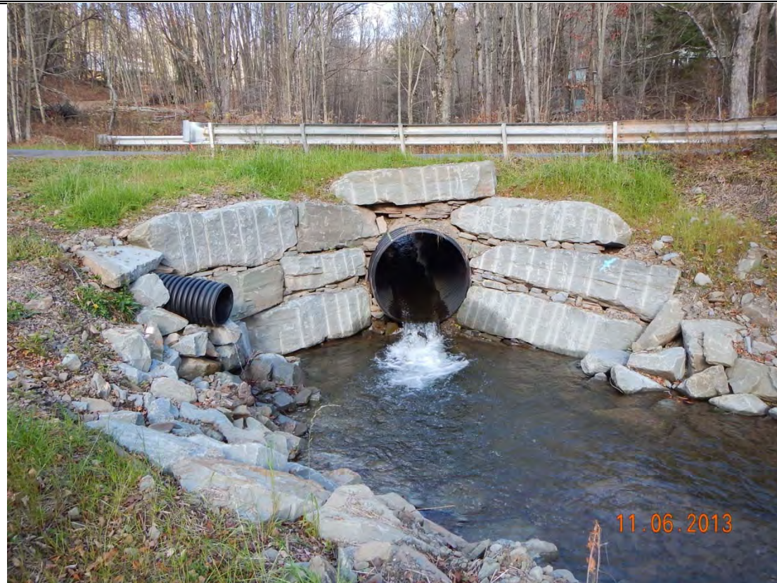
Photo 2: Looking upstream from right streambank at culvert headwall and plunge pool.
