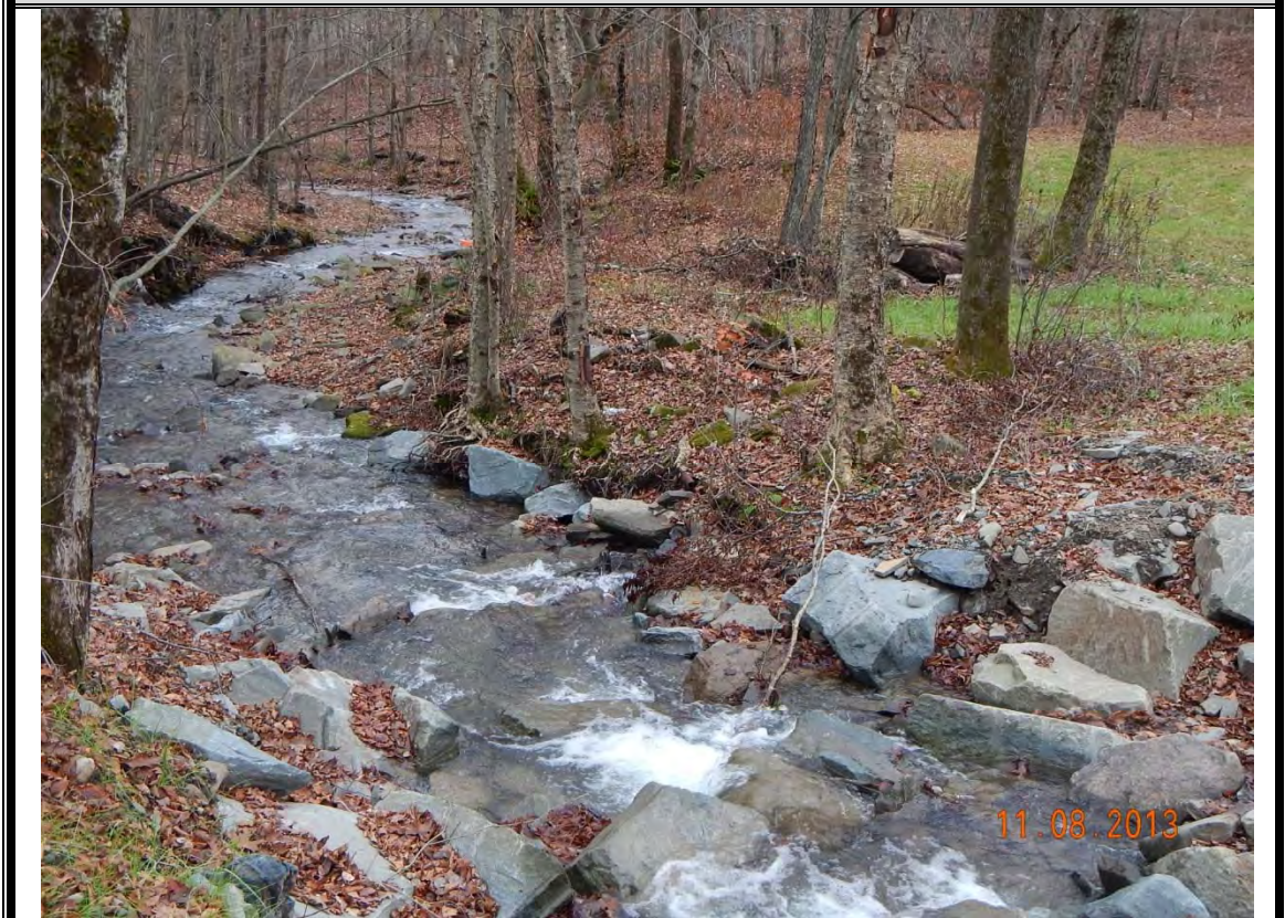
Photo 4: Looking downstream from left streambank after construction of step pool structures.
