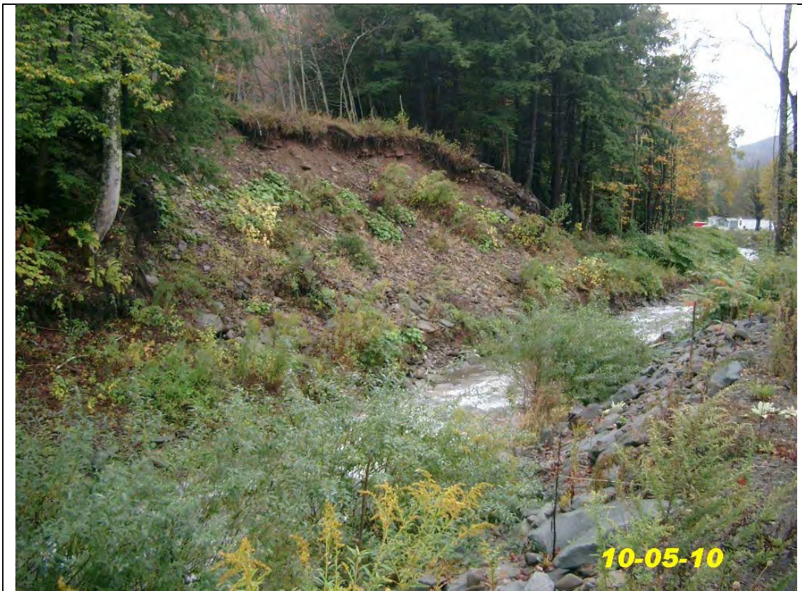
Photo 1: Looking downstream at left streambank erosion from Beers Brook Road.
